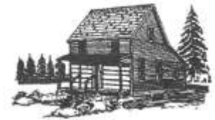
Matsel Cabin East Robinson Street
